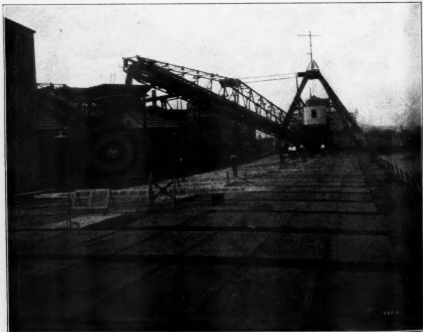
Deck of Freighter Showing Unloading Boom
